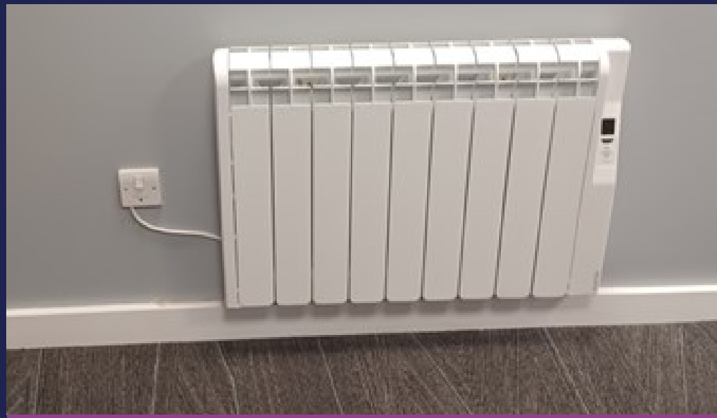
Photo: Wall panel heater replacement
